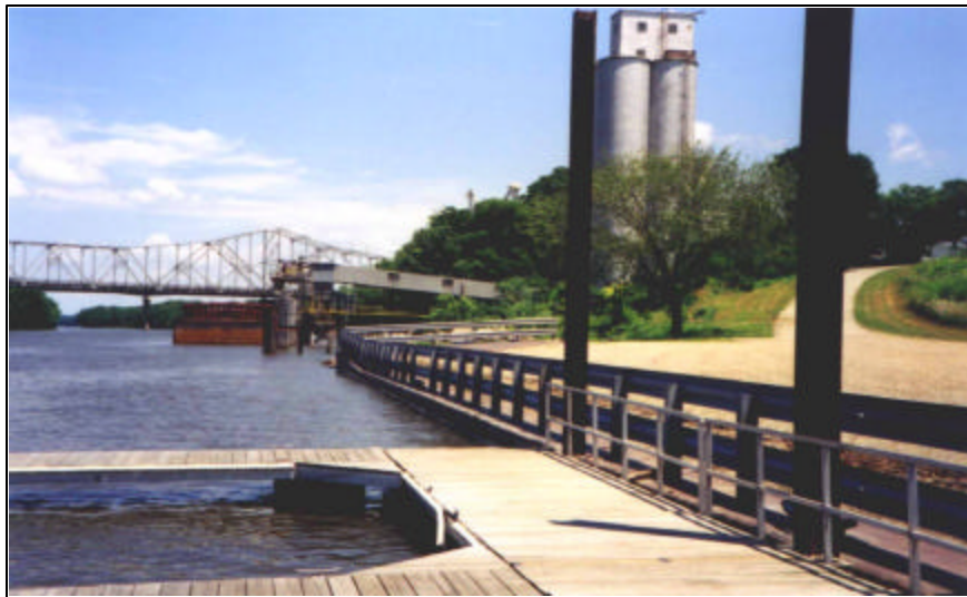
Figure 3.1.7-3 The existing dock in Illinois River at Hennepin.
