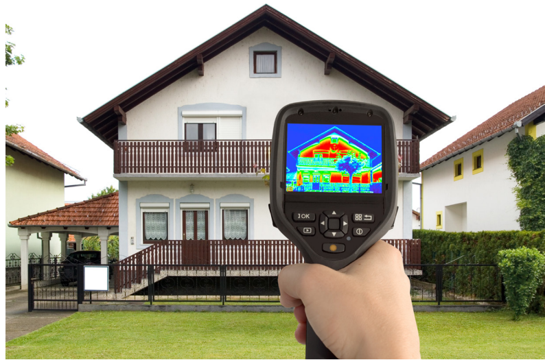
A home's insulation and drafty spots viewed through an infrared camera. Image source: https://www.energy.gov/energysaver/thermographic-inspections
